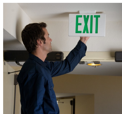
Pay close attention to and maintain public Exit Signs. Make sure they are illuminated.
