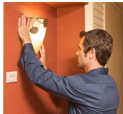
Always be on the lookout for problems with items such as lighting fixtures.
