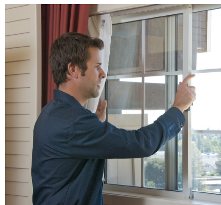
Confirm that windows open and close properly, and that there are no cracks or broken weather seals.
