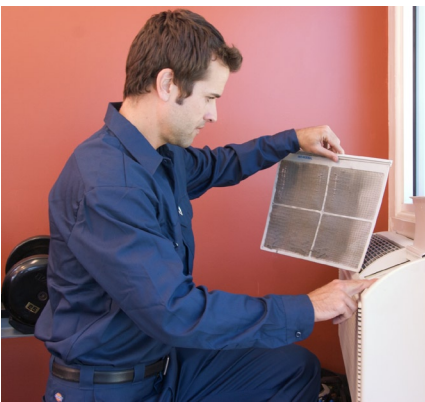
Test the air conditioner to confirm it is working properly and filters are clean.
