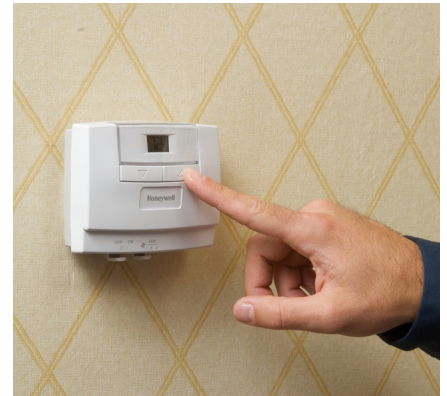
Test the air conditioner heating and cooling controls.
